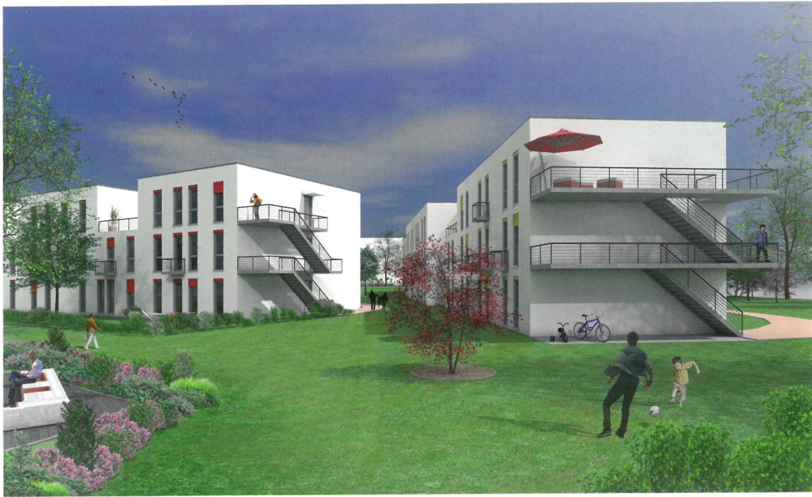
The Havelschanze project envisages modular or serial construction. Optimised, repetitive construction elements shorten construction time and reduce costs. Planning of the buildings using renewable raw materials has already been developed by the Berlin architectural office dgk Architekten. Credit dgk architekten
